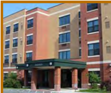
Madison Apartments Built 2011 1000 Madison Street 38 Units
