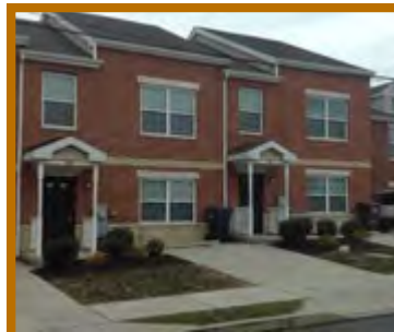
Chatham Terrace Built 2008 611 Central Avenue 48 Units
