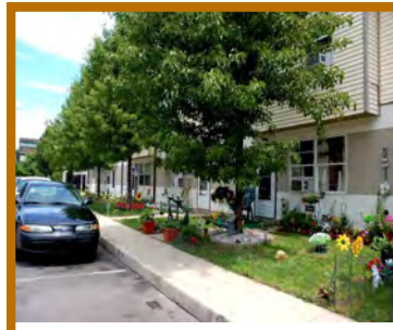
William Penn Homes Built 1942 Rehabilitated 1998 514 Union Street 160 Units
