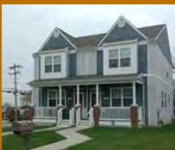
Wellington Heights Built 2012 50 Twin Homes
